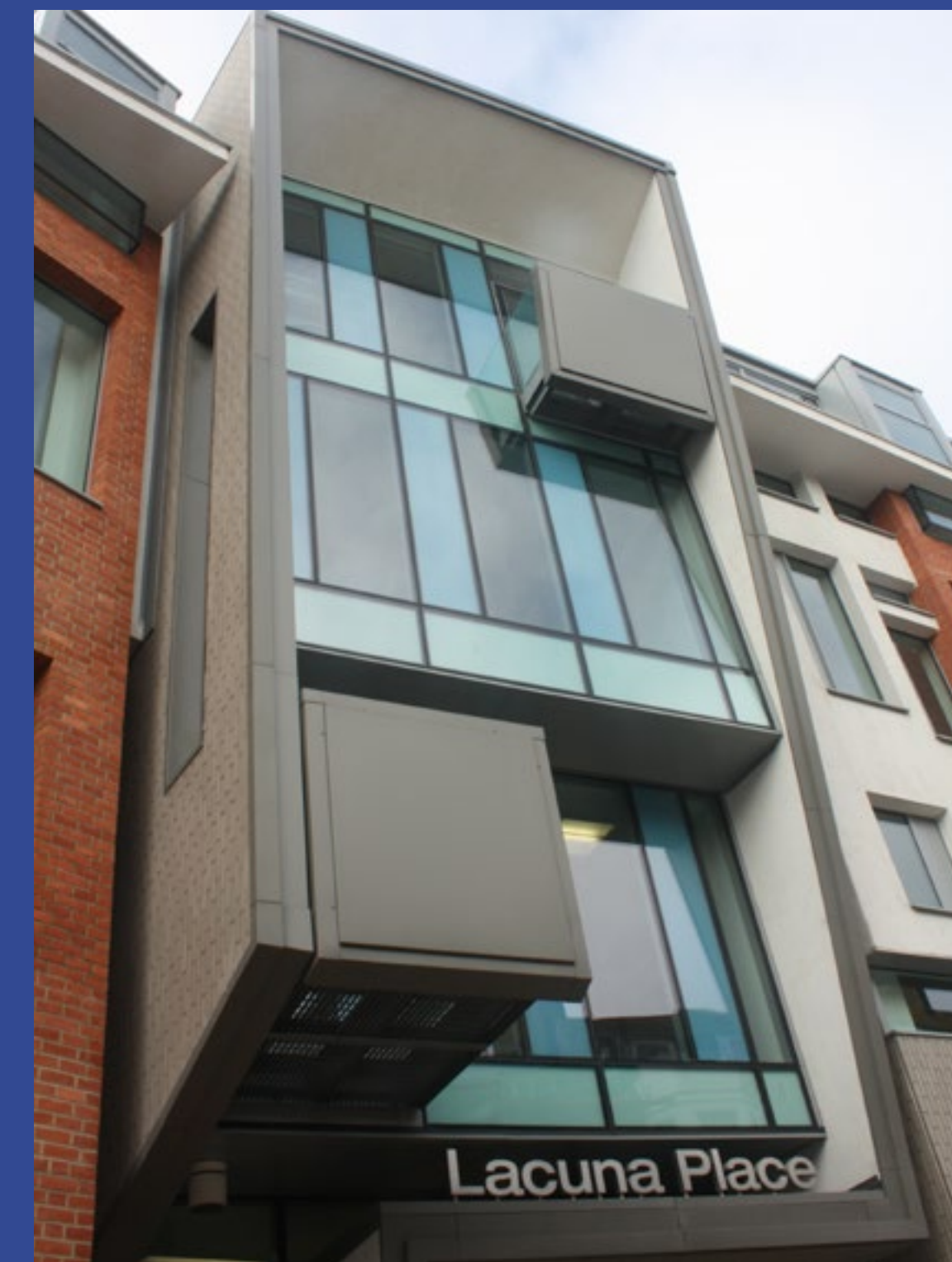
3. Plumpton College (ground floor unit)
