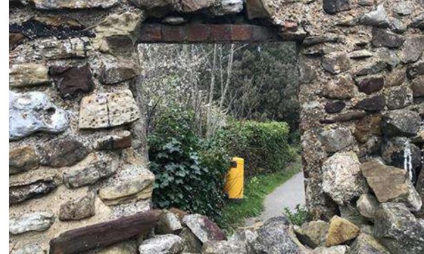
03 | View of existing window aperture at Tea Rooms
