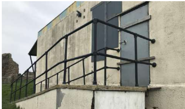
01 | Existing Siege Tent in the castle ground
