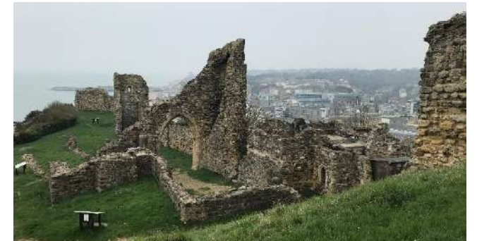
05 | View from the mount inside Hastings Castle
