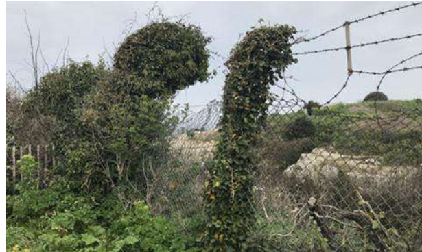
02 | View showing existing concrete post and wire fencing
