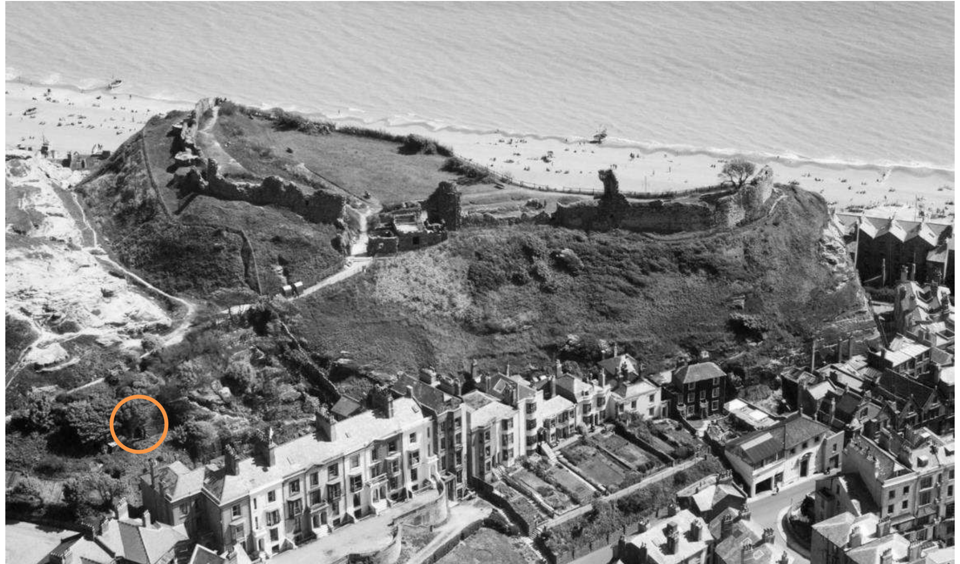
Figure 4.2. - Aerial Photo - EAW006148 (Historic England)
